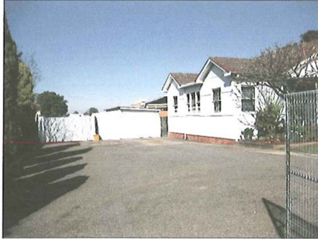
Photograph 2: Subject Site No.131 Polding St
