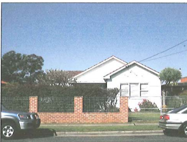
Photograph 1: Subject Site (No.131 Polding St) viewed from across the road looking south
