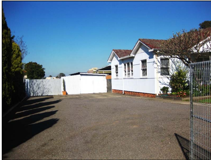
Photograph 2: Subject Site No.131 Polding St
